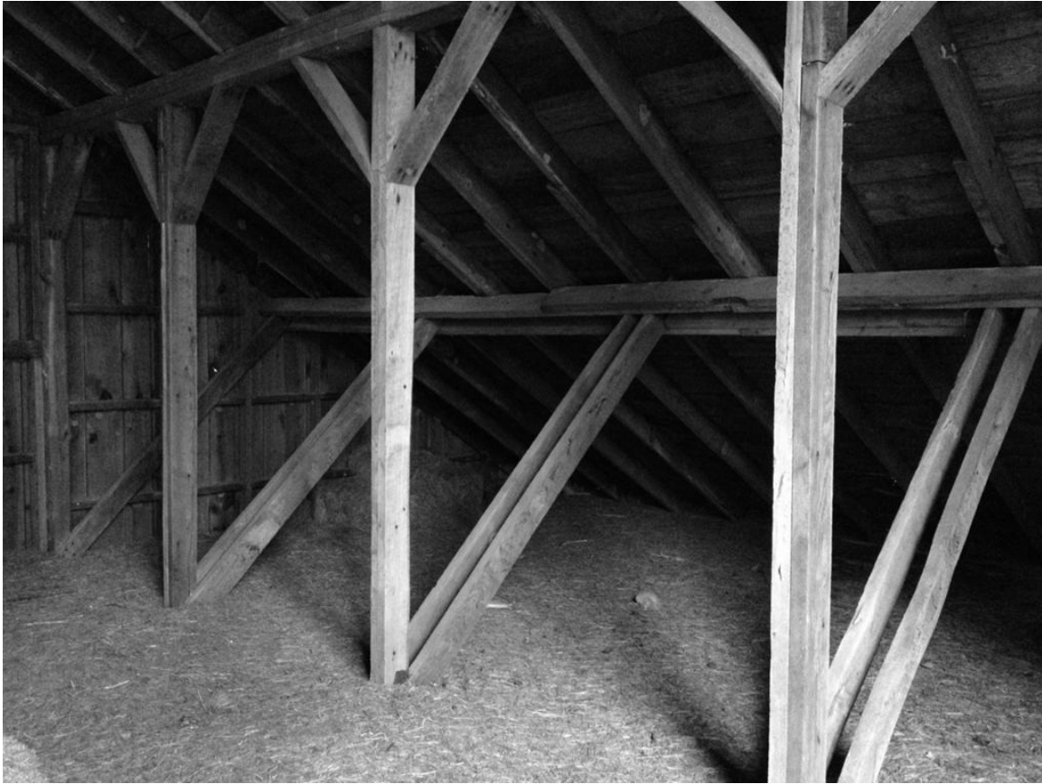
VA_Orange County_Montpelier Sheep Barn_Gang Planking in Hay Loft.jpeg
