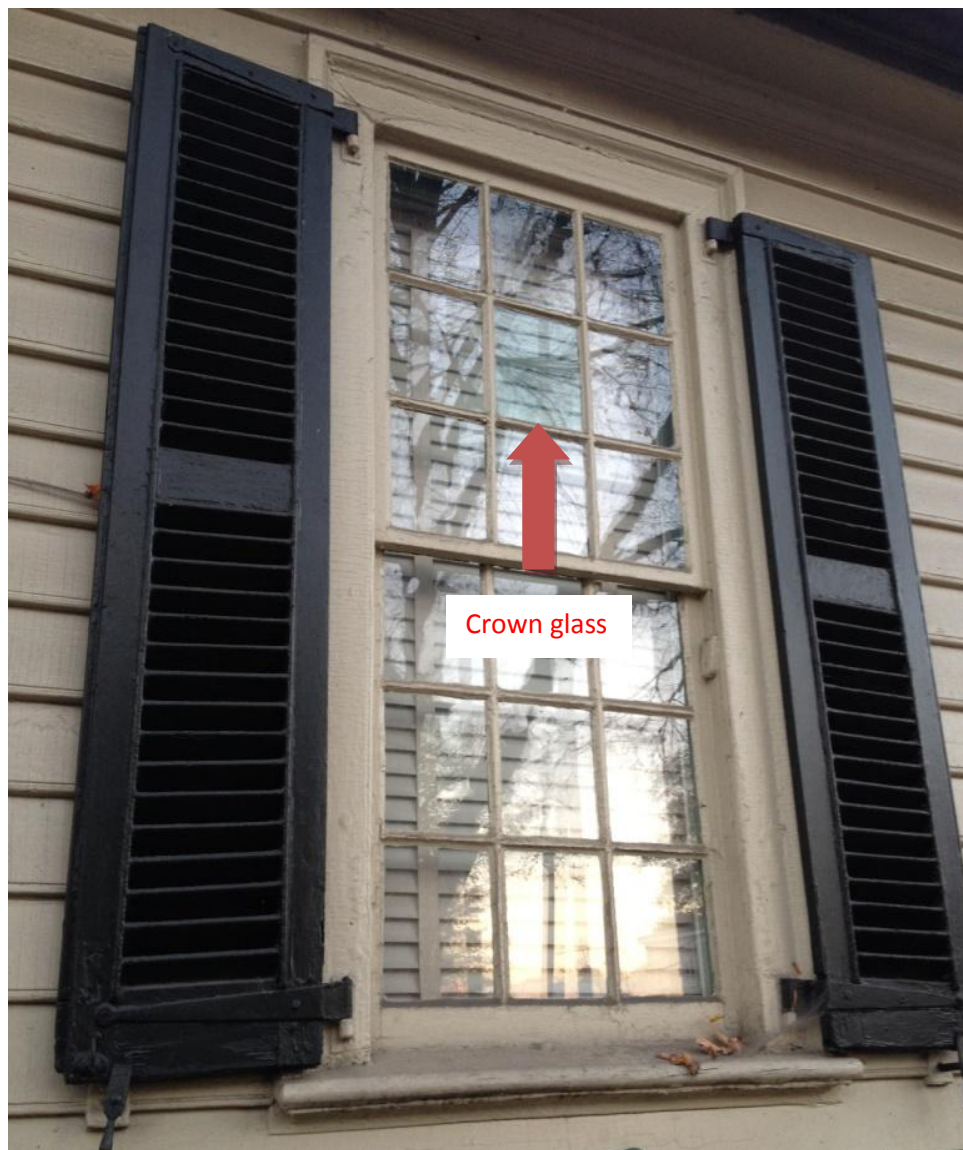
Figure 14: This window primarily has cylinder glass. The blue tinted pane is crown glass.
