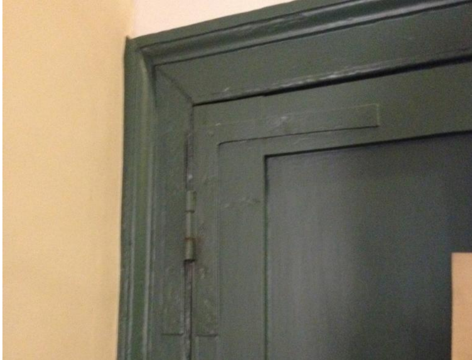
Figure 17 shows an HL hinge.
