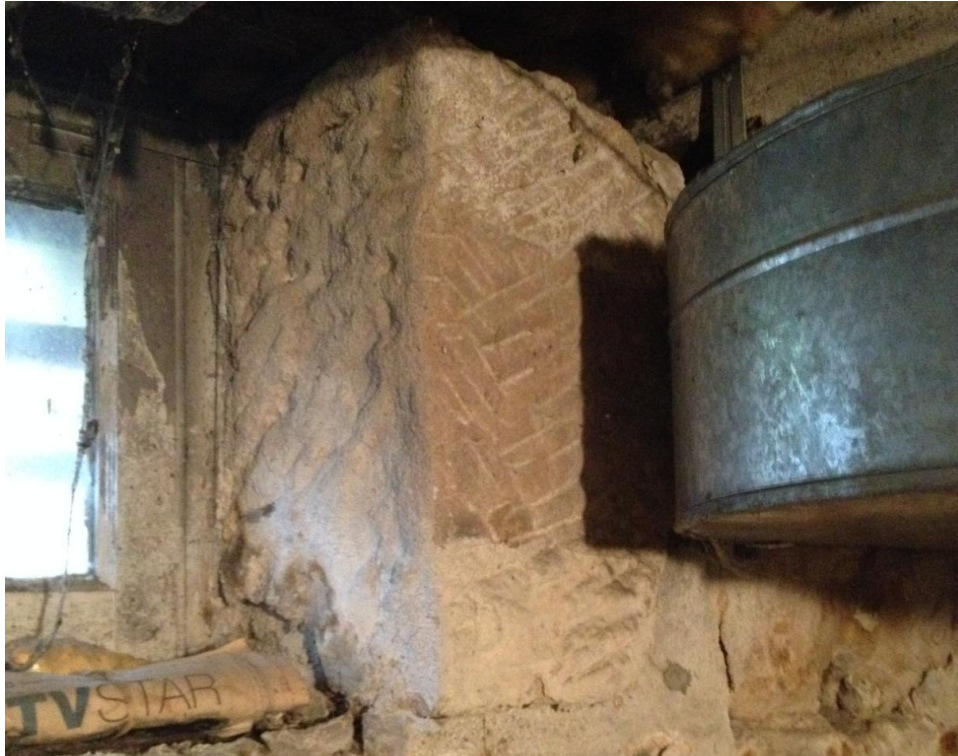
Figure 7 shows the scabbed Aquia sandstone.
