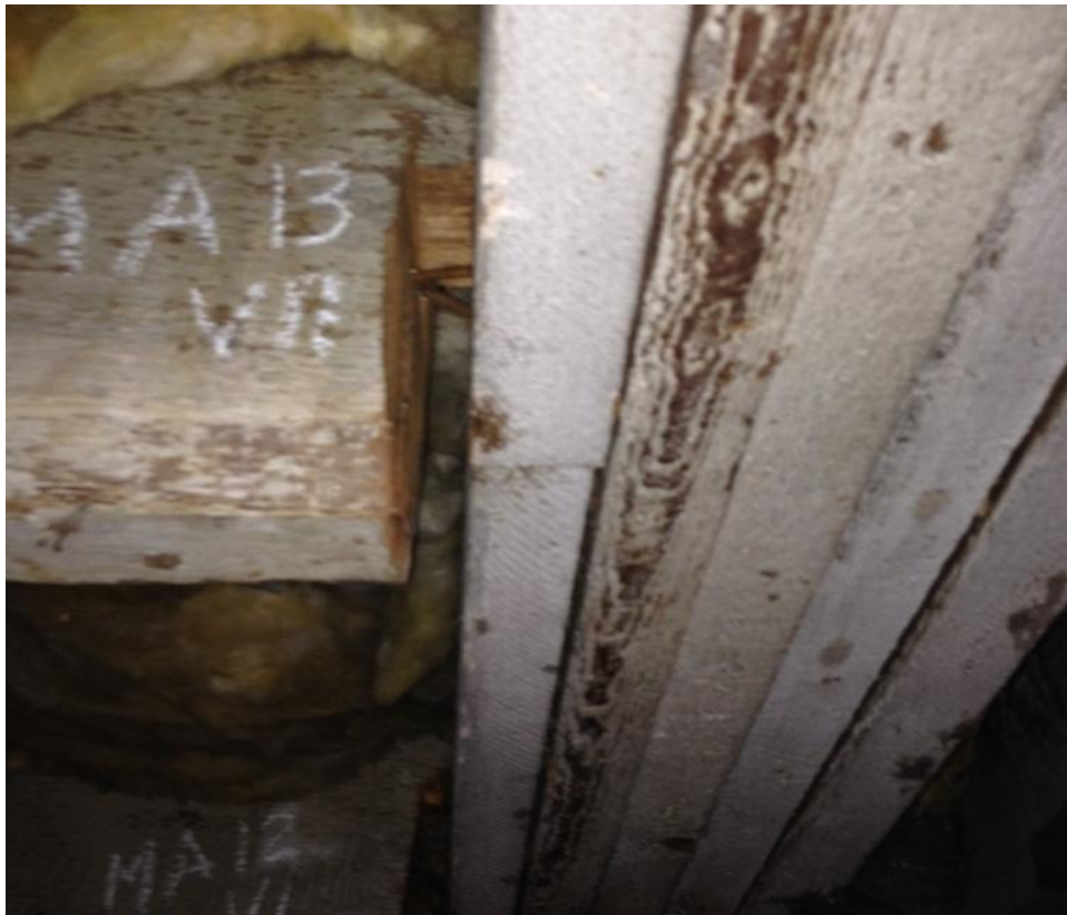
Figure 3 shows the summer beam comprised of gang planked and circular sawn lumber.
