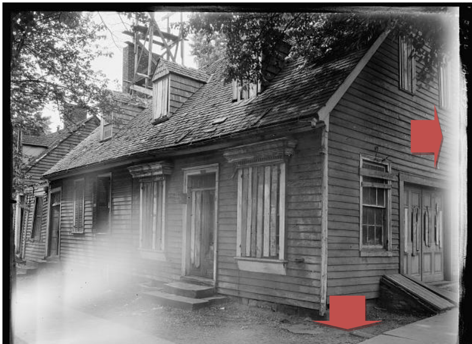
Figure 8: This photograph by Frances Benjamin Johnston shows the original location of the bulkhead, as well as the access doors.
