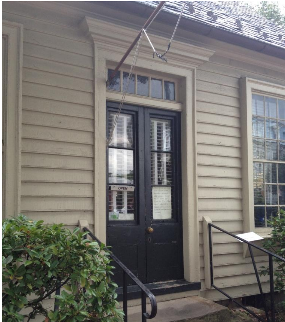
Figure 16: The buildings glazed doors with this type of doorknob do not date to the building's period of significance. The pediment above the door is also not original.
