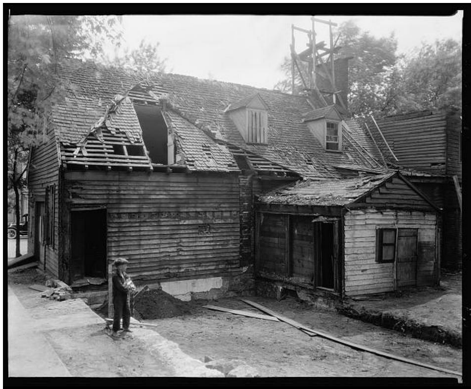
Figure 8: This photograph by Frances Benjamin Johnston shows the site of the one-and-a-half story buildings, as well as the ongoing demolition of the two-story building. The image also shows the original wood shingles as well as the door that connected the shop to the lumber/compting house. (Image from the Carnegie Survey of the Architecture of the South Collection at the Library of Congress)
