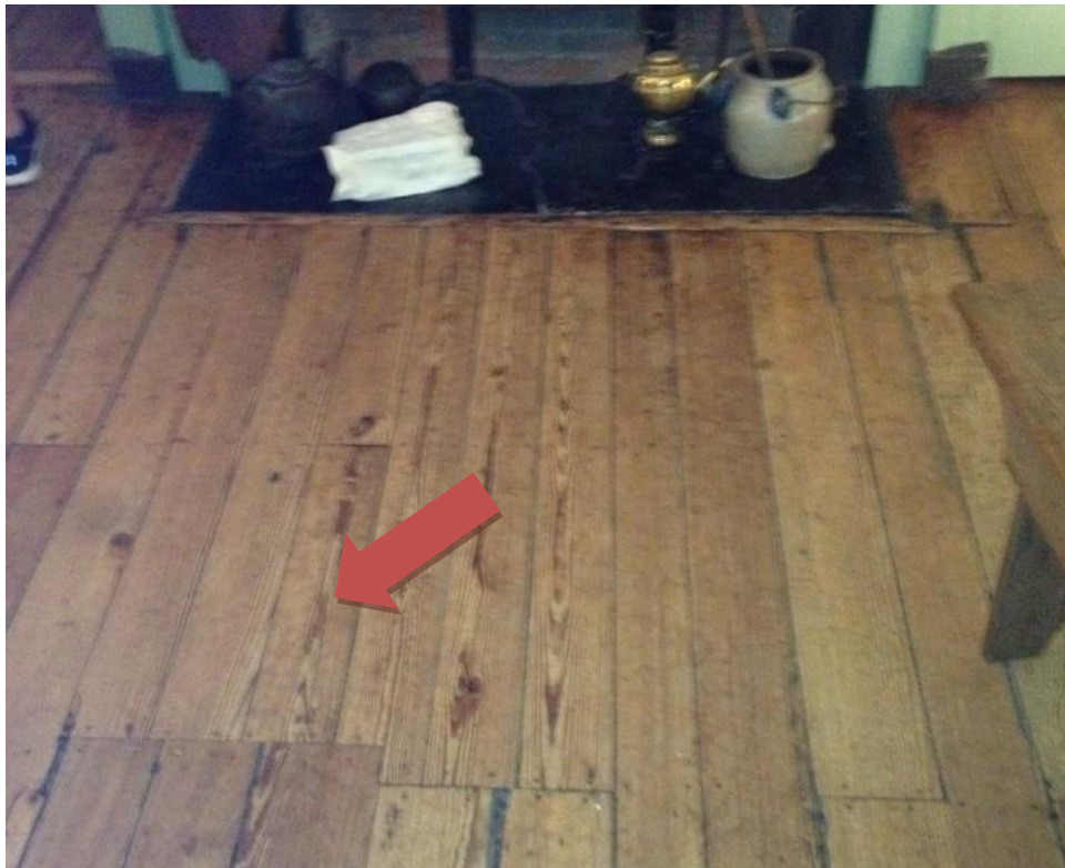
Figure 18 shows where the flooring has been altered in the southeast room.
