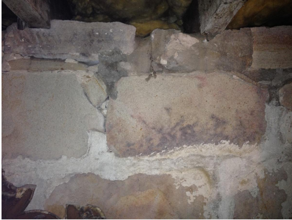
Figure 6 shows Portland mortar repairs.
