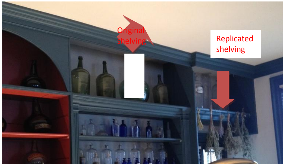
Figure 22: The shelving at the end was based on the original shelving in the center. Again, the new shelves have sharper molding profiles than the originals.
