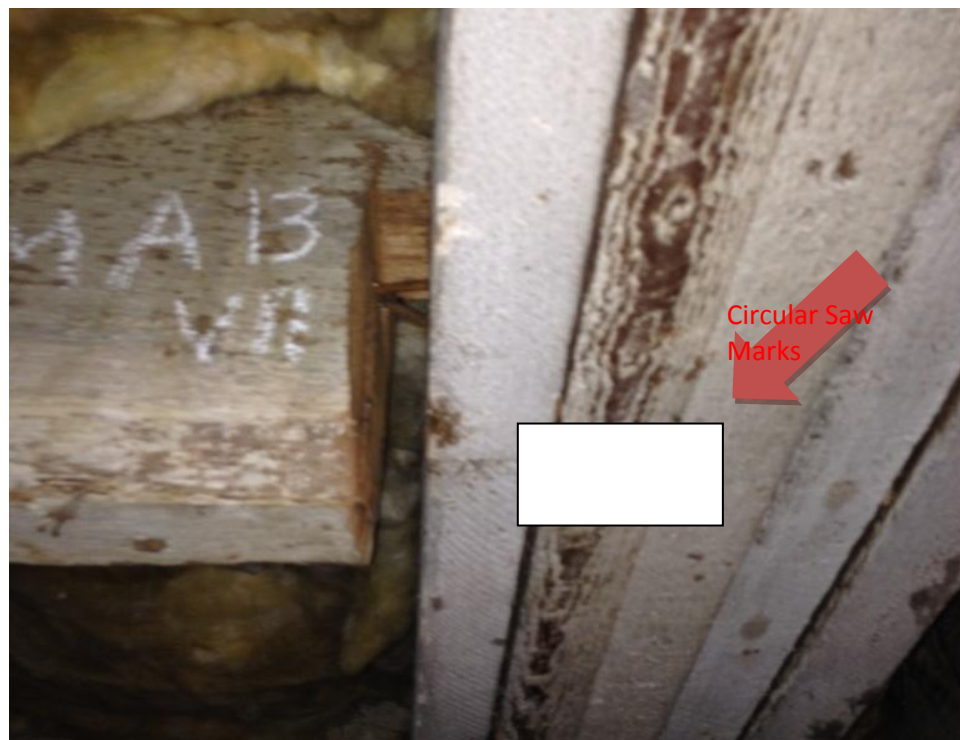
Figure 12 shows the circular sawn, gang planked summer beam.
