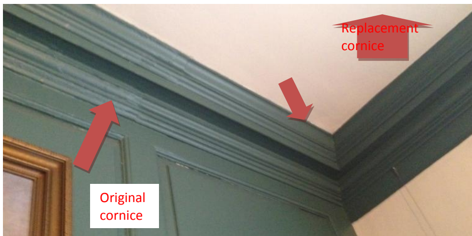
Figure 21 shows a section of cornice that has been replaced. The original cornice has muted edges from numerous layers of paint, while the replacement cornice has sharper edges.
