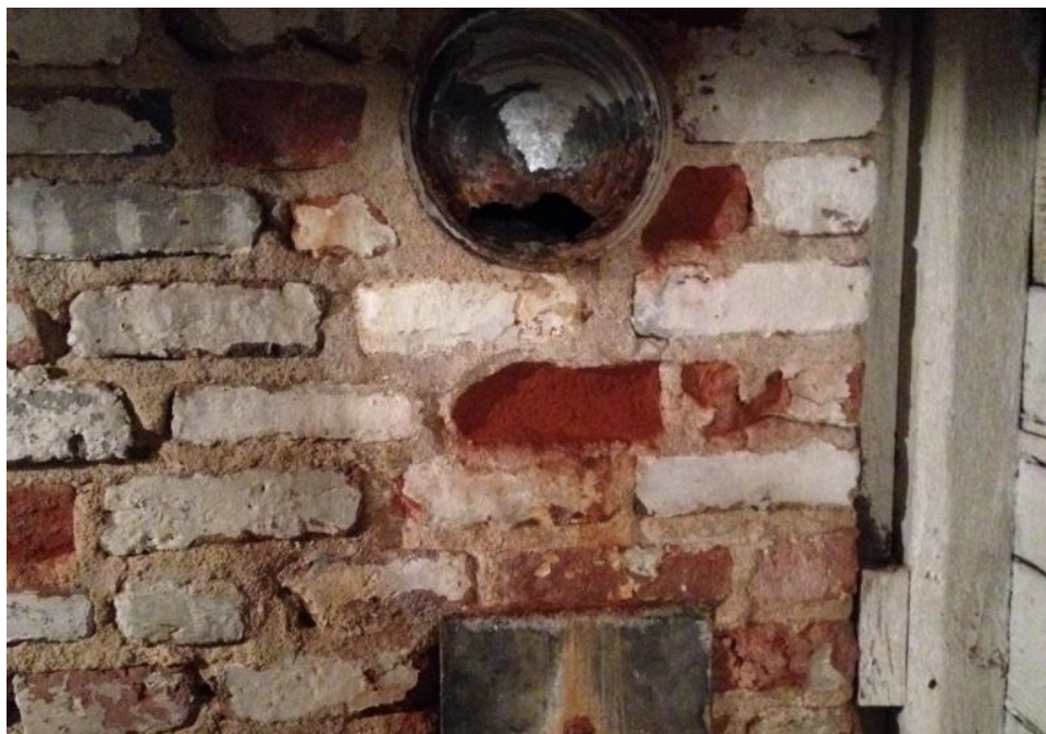
Figure 10 shows the hard edges and fewer irregularities of machine pressed brick.
