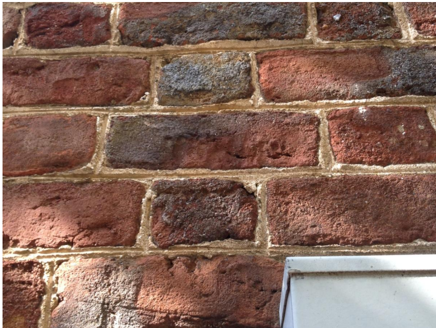
Figure 5 shows the hand pressed brick with finger prints.
