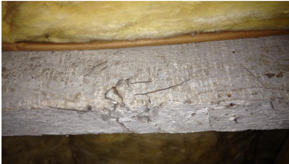
Figure 2 shows a hewn and pit sawn joist.
