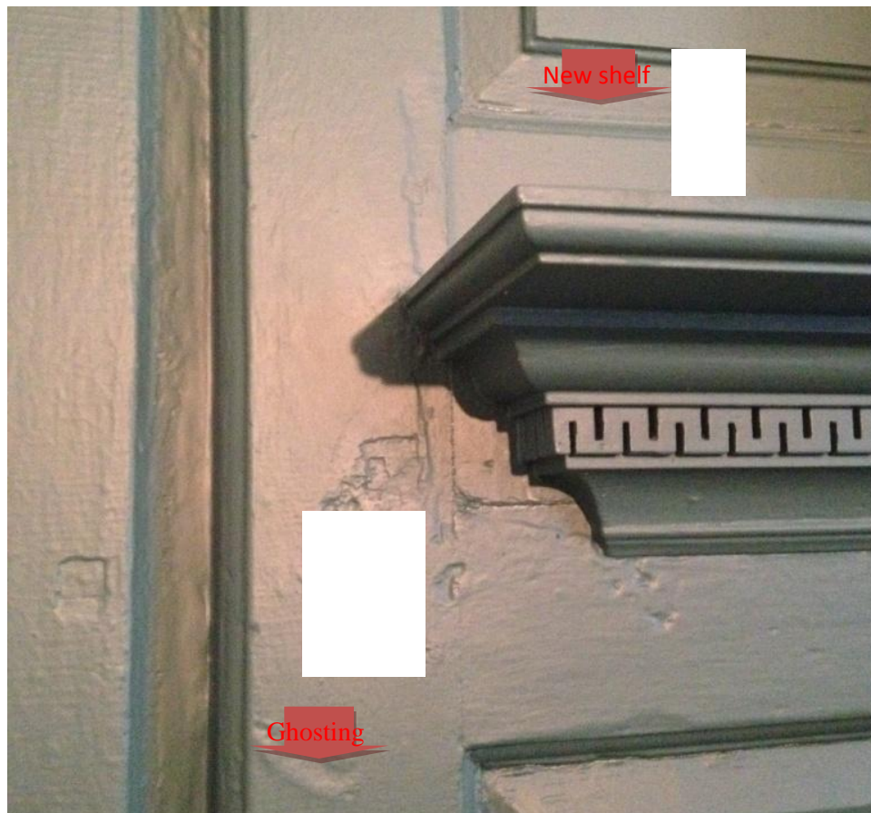
Figure 23 shows ghosting where features have been removed from the mantelpiece. The fretwork shelf is a newer feature that does not date to the building's period of significance.
