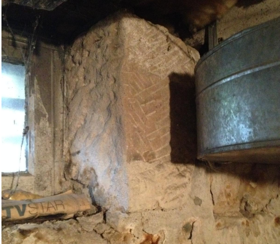
Figure 4 shows the scabbed Aquia sandstone.
