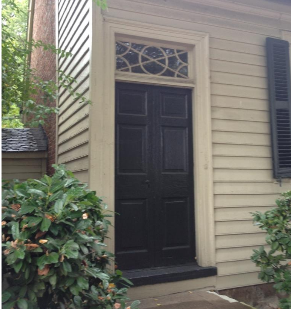
Figure 15: Six panel doors (or double doors in this example) with deep paneling date to the building's period of significance.
