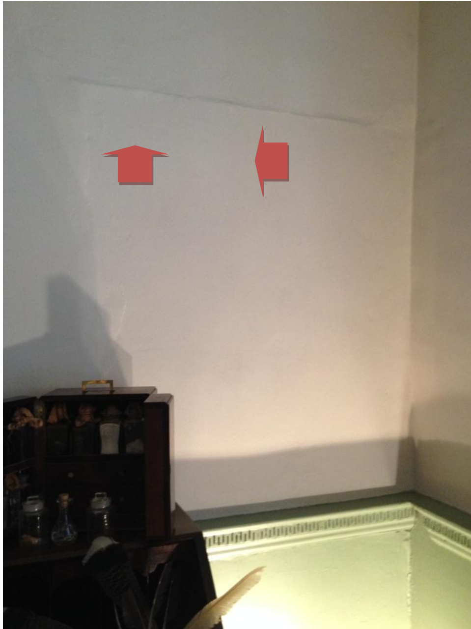
Figure 19 shows where the doorway used to be between the shop and the dwelling.
