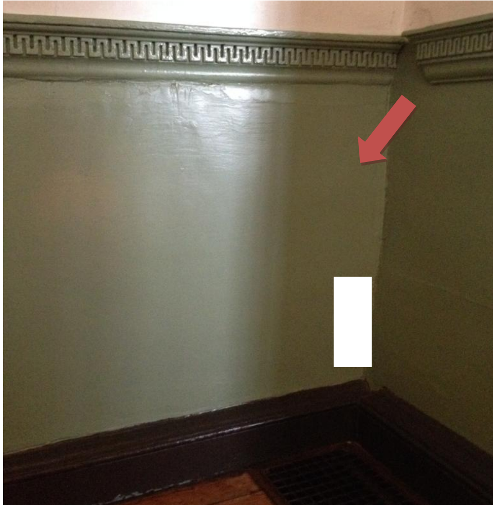
Figure 20: Irregularities in the junction of the mopboard and the chair rail show where the entrance to the basement stairs used to be.
